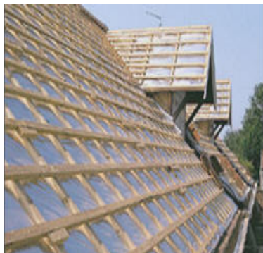
TRI-ISO SUPER 10 Installed prior to fitting roof tiles
